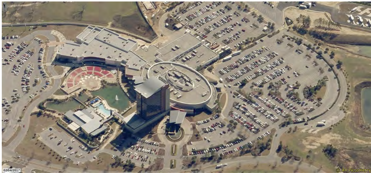
WIND CREEK CASINO, ATMORE
